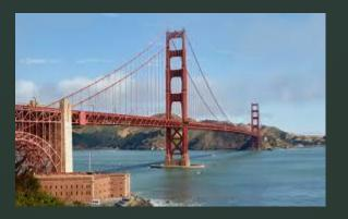
**The Golden Gate Bridge:-** It is a suspension bridge of total length 2.74 km (8980 ft). The span distance of this bridge is about 4200 ft . It is famous as one of the world's most beautiful bridge.
